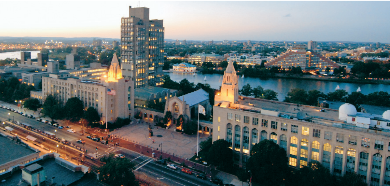
MARSH CHAPEL, FLANKED BY THE ORIGINAL MAIN BUILDINGS ALONG COMMONWEALTH AVENUE.
